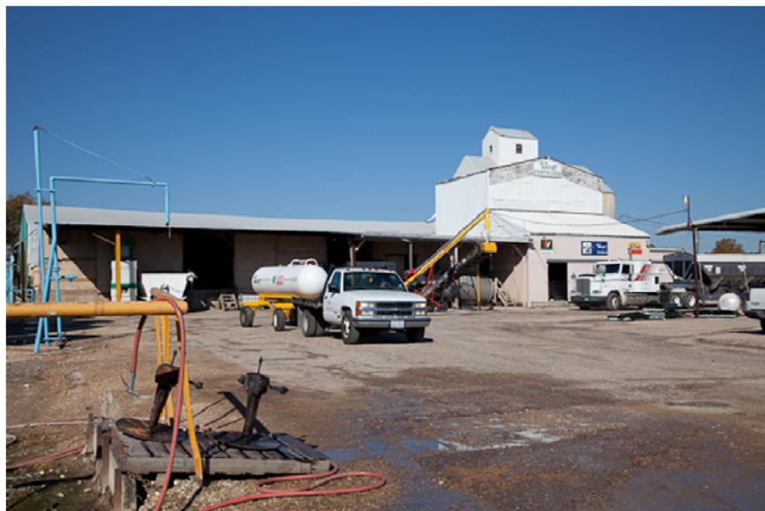
East side of the processing building where the mixing and delivery of chemicals occurred
