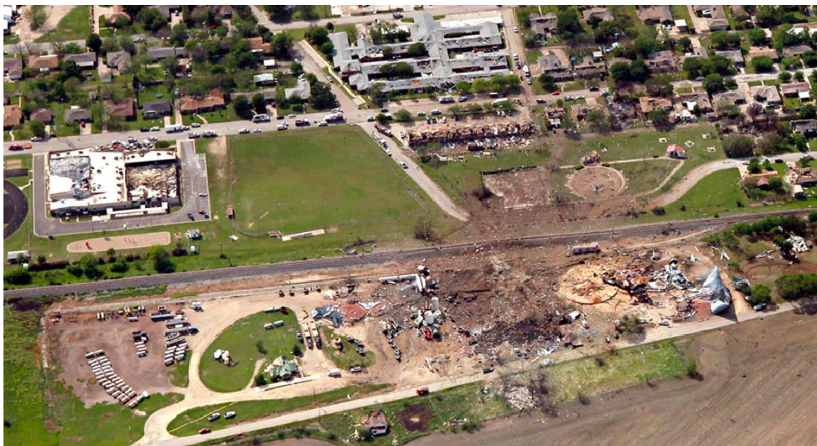
View of the site prior to scene excavation and examination
