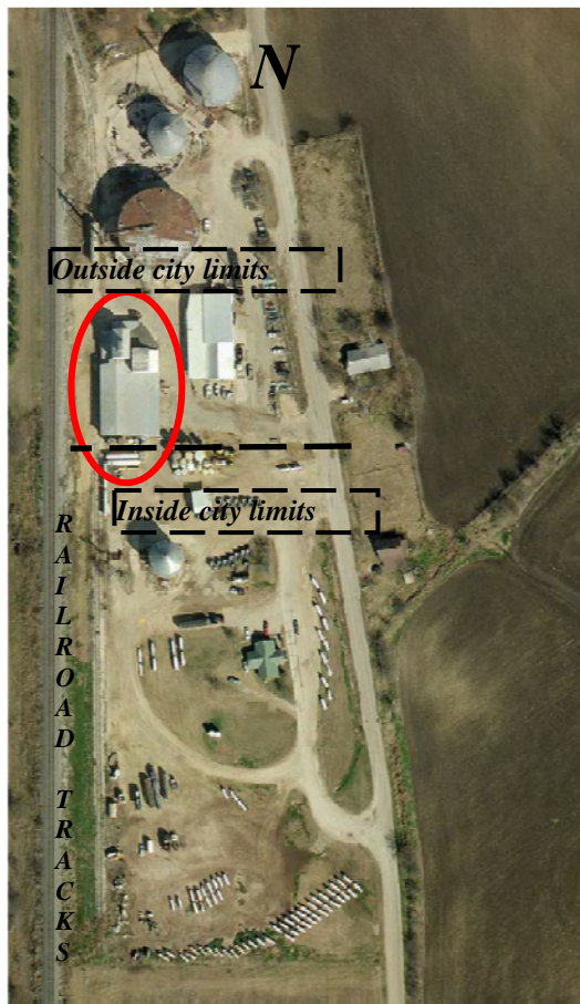
West Fertilizer showing the city limits, the processing building (red circle), and railroad tracks
