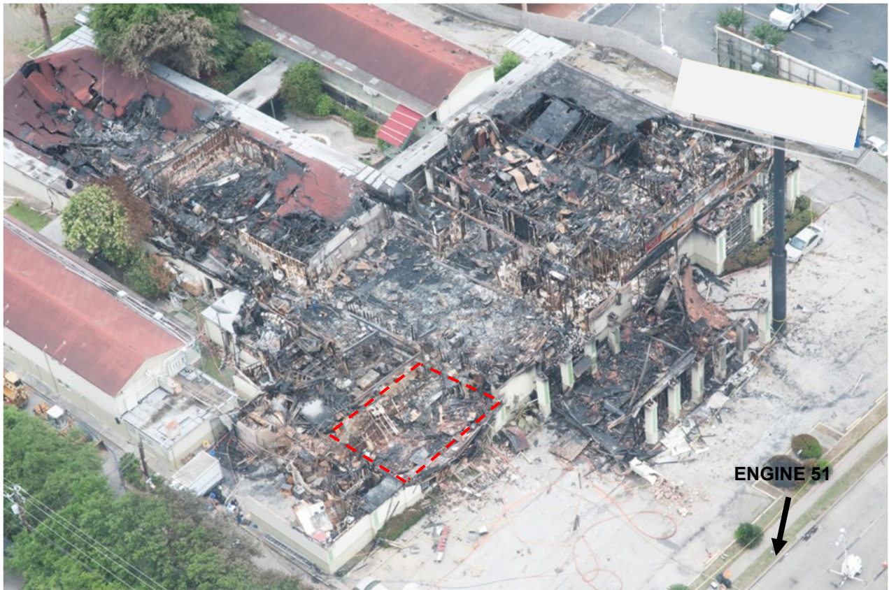
Banquet room area of roof collapse
